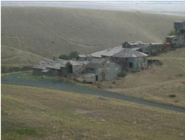
Mine Complex near Silver Star, MT
