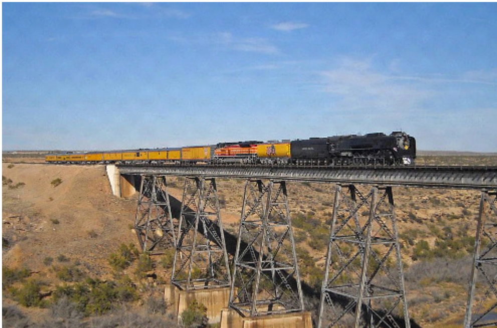
UPRR 844 pulling the Centennial Special crossing bridge near Logan, NN on November 4, 2011.
