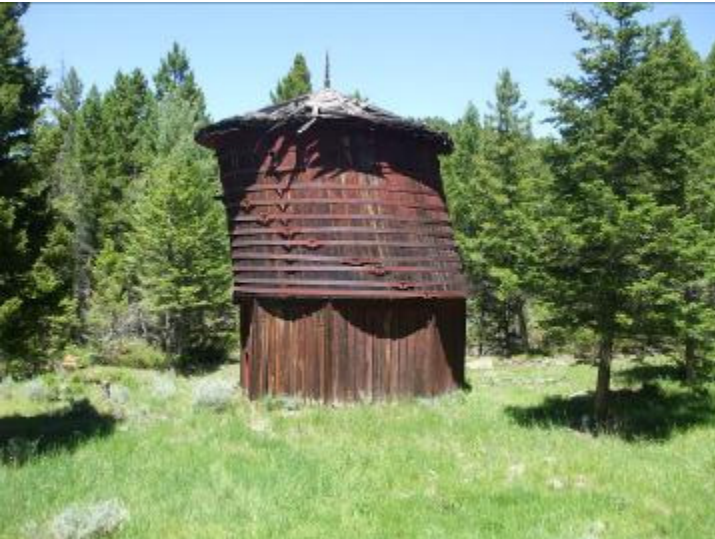
Northern Pacific water tank in Elkhorn, MT
